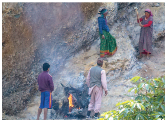
Photo 7: Hard rock sections are heated by a fire and become brittle after cooling down over night
