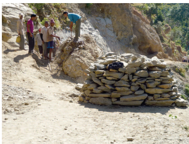
Photo 8: Excavated stones are stored and reused to construct protective structures
