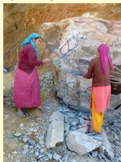
Photo 4: Women gained confidence during road construction
