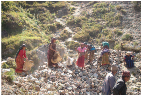
Photo 3: Collection of stones for preparation of gabions
