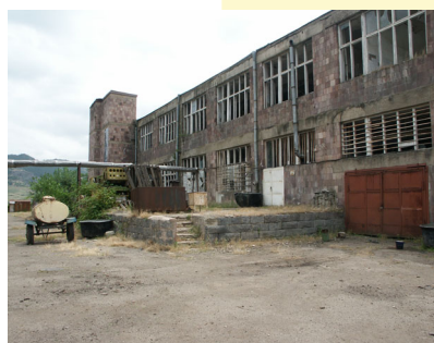
Picture 2: Industry and infrastructure needing rehabilitation
