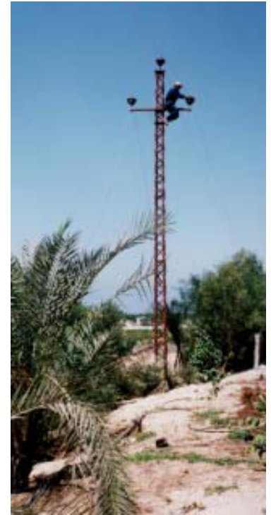
Photo 1: Tension lines are being mounted to the electricity poles
